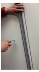
7. Swing the height rod channel back to its vertical position. Align the four screw holes with the inserted drywall anchors or drilled lead holes and insert the remaining four 1-1/4" screws. Tighten all screws, including the top screw, until height rod is held firmly against the wall.
