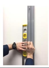
Swing the height rod channel to the side to drill lead holes into the marked locations. If mounting to drywall or plasterboard, obtain the four remaining drywall anchors and using a Phillips head screwdriver, insert the anchors into the wall.
