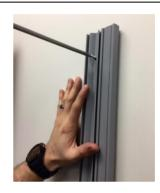
5. Using a level, make sure the height rod channel is plumb/straight. Mark the remaining four holes.
