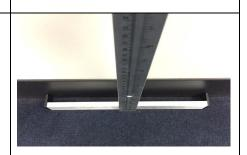
Use a level to ensure the height rod is vertically straight and plumb. While holding the level and height rod in place, insert a thin pencil or screw to mark the screw hole in the top hole. Next mark the screw holes for the center and bottom holes.
